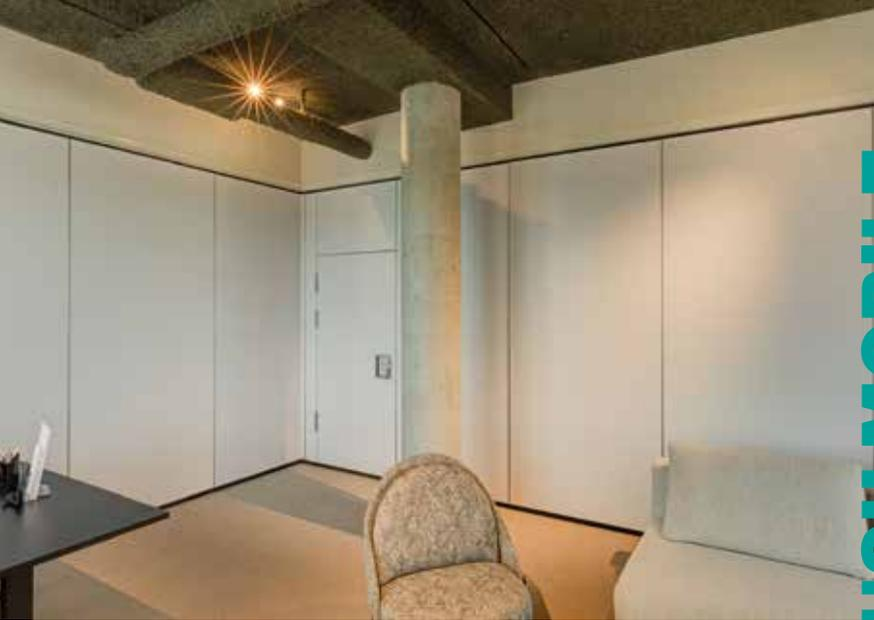
**Movable or operable partition wall supported on tracks from above without any floor tracks.**
